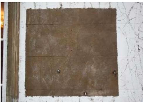
Removal of 25 year old alkyd based masonry paint and primer from Portland Cement based render using Restorative Polyurethane Softener. Residue rinsed with the ThermaTech® system.
