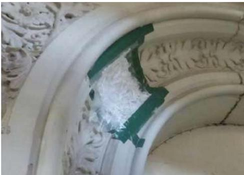
A test area has been prepared using an application of Restorative Polyurethane Softener. The paint coatings are very thick and the prevailing temperatures cold so the softener was applied thickly and the sample covered with tape and polythene and left for several days. The formulation has a slow evaporation and so has a wide 'window of removal'.
