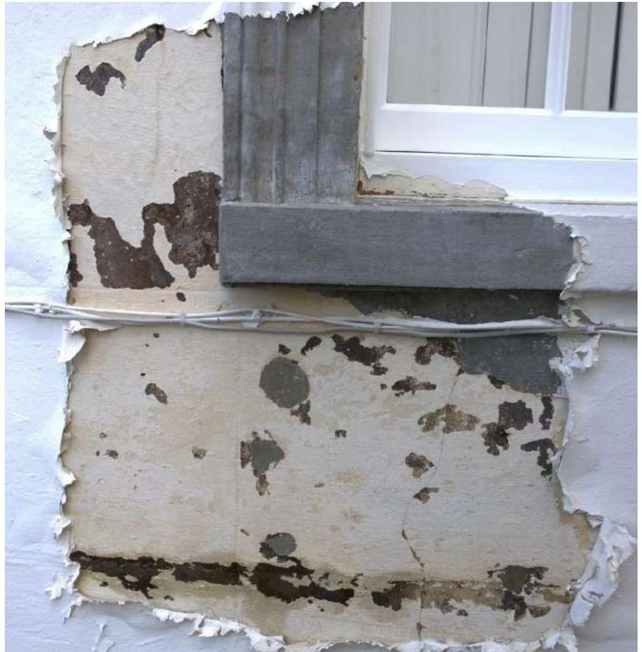
Photo above: Multiple layers of acrylic and other thermoplastic masonry paint removed with a ThermaTech system. This has exposed a proprietary cement based paint (Snowcem or similar). The removal has also revealed some cracking and Portland cement repair to the Roman Cement stucco. In this case a silicate based mineral paint was selected as the replacement. This will normally adhere well to mineral substrates including cement based paint negating need for further removal.
