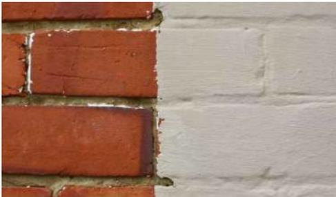
Removal of alkyd masonry paint using Restorative Polyurethane Softener exposing 'Snowcem' type cement based masonry paint. The Snowcem dissolved using Restorative Cement Based Paint/ Lime Remover. Residue rinsed with the ThermaTech® system.
