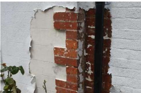
Removal of acrylic based paint from brickwork and Snowcem painted stucco. No chemical treatment required. Some lime paint remaining to brickwork that can be removed by careful scraping.
