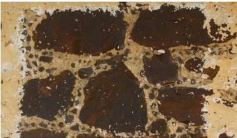
Removal of Snowcem type coatings from Ironstone, flint and limework masonry.
