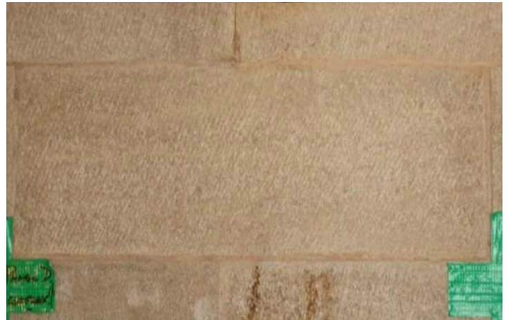
Removal of tannin and water staining from internal stonework – second photo taken 72 hours after cleaning.
