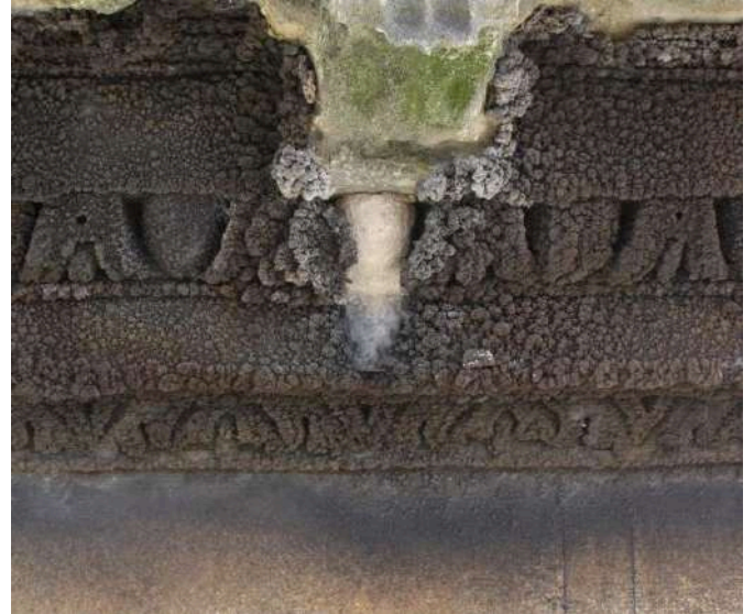
Carbon Sulphation may accumulate in thickness from a film, to a 'clinker' of several centimetres
